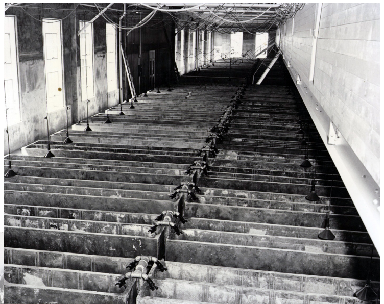
Concrete nursery troughs in place. May 9, 1940.
