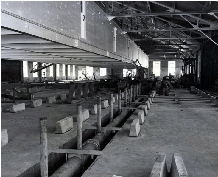
Loft walled in, trough supports and pipes in progress. March 12, 1940.
