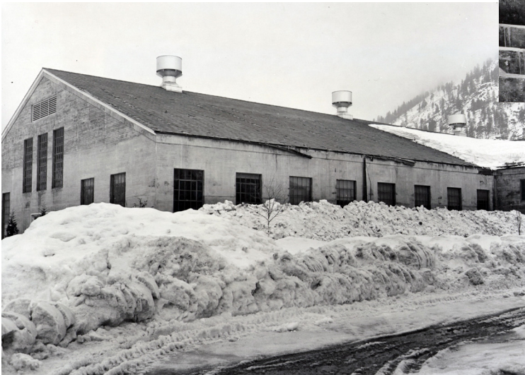
Original gutters torn loose by sliding snow. February 16, 1943.
